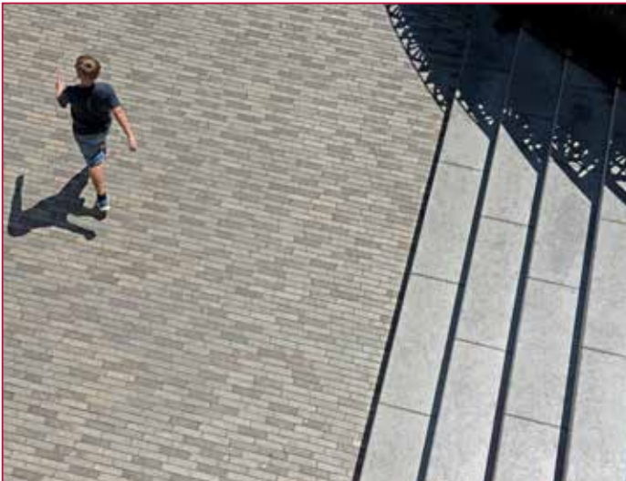
Fertige Verfugung aus der Vogelperspektive | Bird's eye view of finished joints
